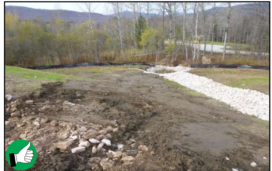
After installing rock outlet protection
