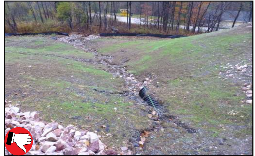
Before installing rock outlet protection
