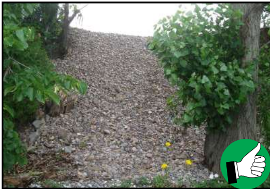
Stone rip-rap installed on an unstable slope with a stormwater outlet pipe along the slope.
