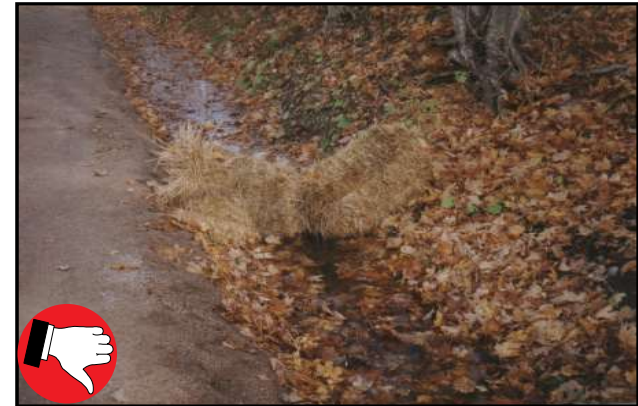
Hay bales must not be used as check dams due to their high failure rates.
