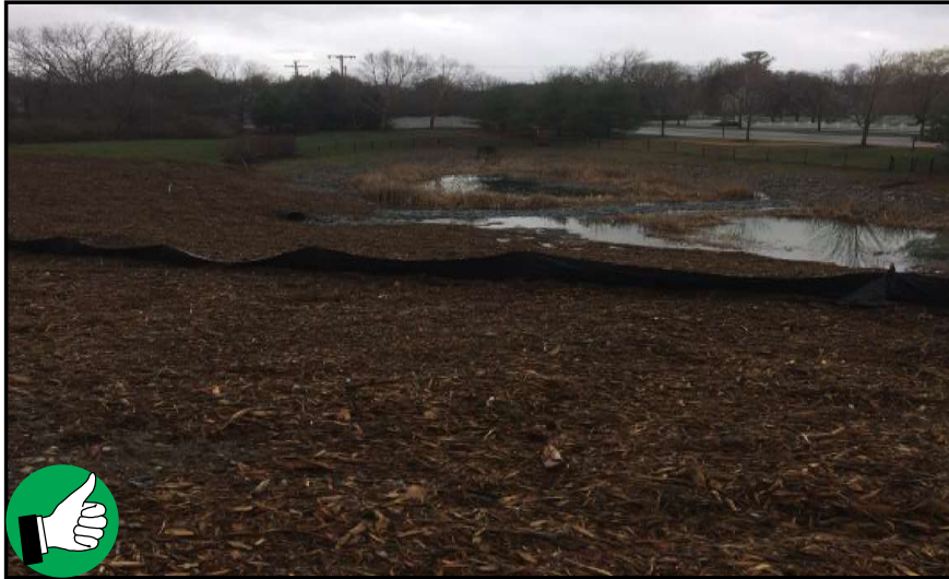
Good application of wood chip mulch and stump grindings.
