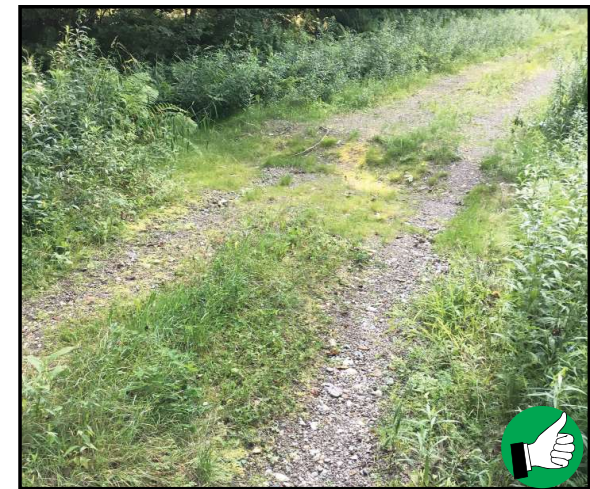
Good installation of a water bar along an access road.
