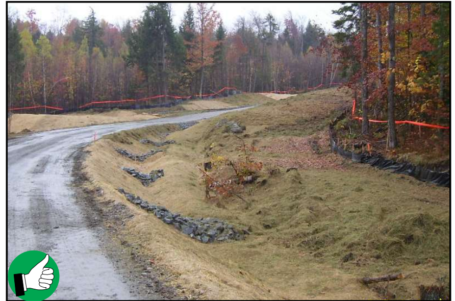
Good installation of rock check dams. The check dams should extend up the sides of the banks. Middle section should be lower than the sides. Clean out sediment as it accumulates.
