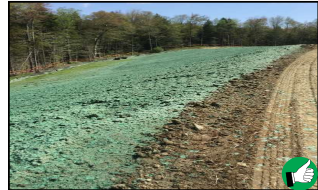
Excellent application of hydroseed with a mulch component. Entire soil surface has been covered and is temporarily stabilized.
