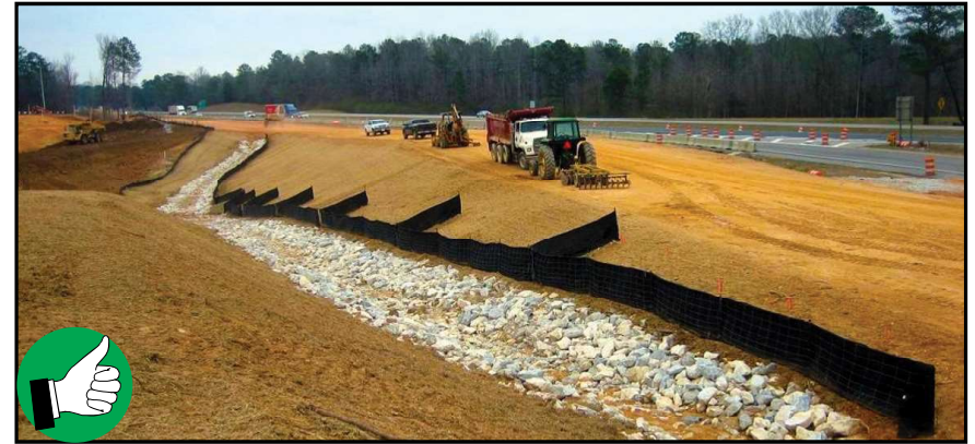
Excellent installation of reinforced silt fence and j-hooks in front of a stone-lined drainage channel.
