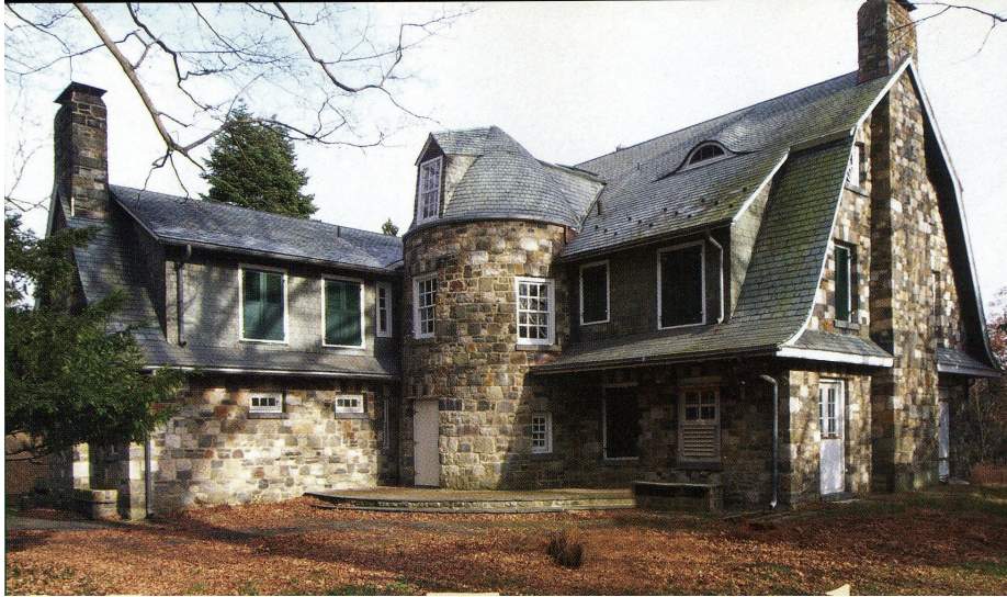
Note the lack of visible equipment outside the 1912 Marie Zimmerman House in Bushkill, PA. Use of geothermal eliminated aesthetic intrusions on the facades of this historic house.
