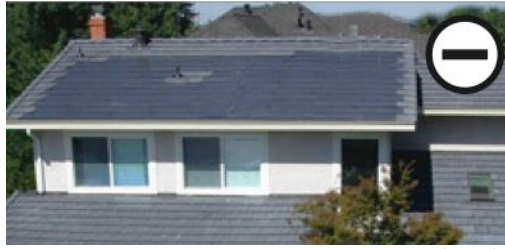
City of Santa Barbara, Solar Energy System Design Guidelines (2006) pg. 21
