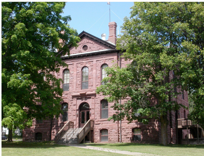
The original Bayfield County Courthouse has been rehabilitated to provide a Headquarters and Visitors' Center for the Apostle Islands National Lakeshore. Photo: V. Birenberg
