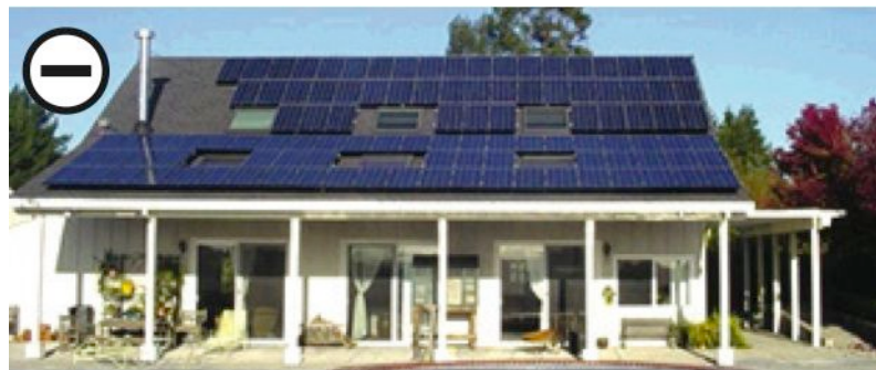
All photos from City of Santa Barbara, Solar Energy System Design Guidelines (2006), p. 25.
