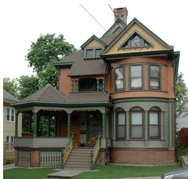
The use of dark paint schemes on Victorian-era buildings maximized solar heat gains in the winter in cold climates. Photo courtesy of Neal Vogel.
