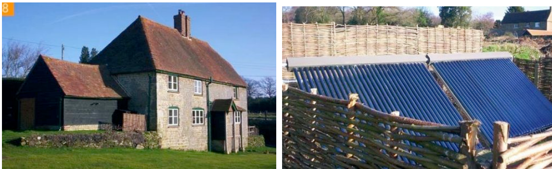
Solar thermal installation in West Sussex, England on a National Trust cottage dating to the 17 th century. The small willow fence next to the cottage screens the collector. Photos by Robert Williams. English Heritage, Small-Scale Solar Thermal Energy and Traditional Buildings , (2008), p.7.
