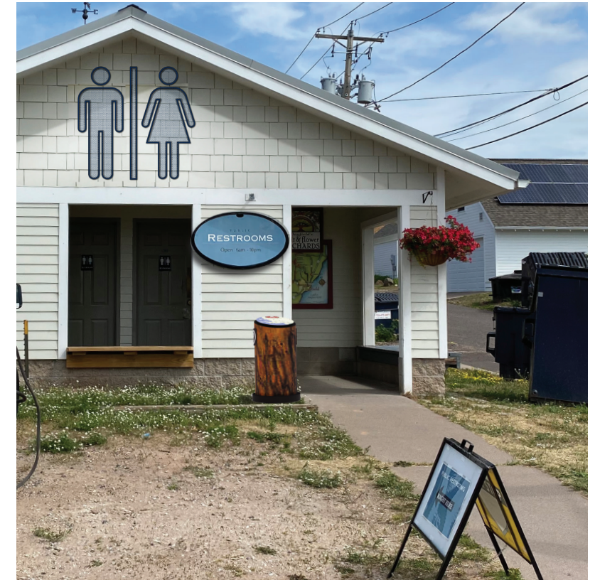
3 Photo Composite SCALE: NTS Maypenney Restrooms
