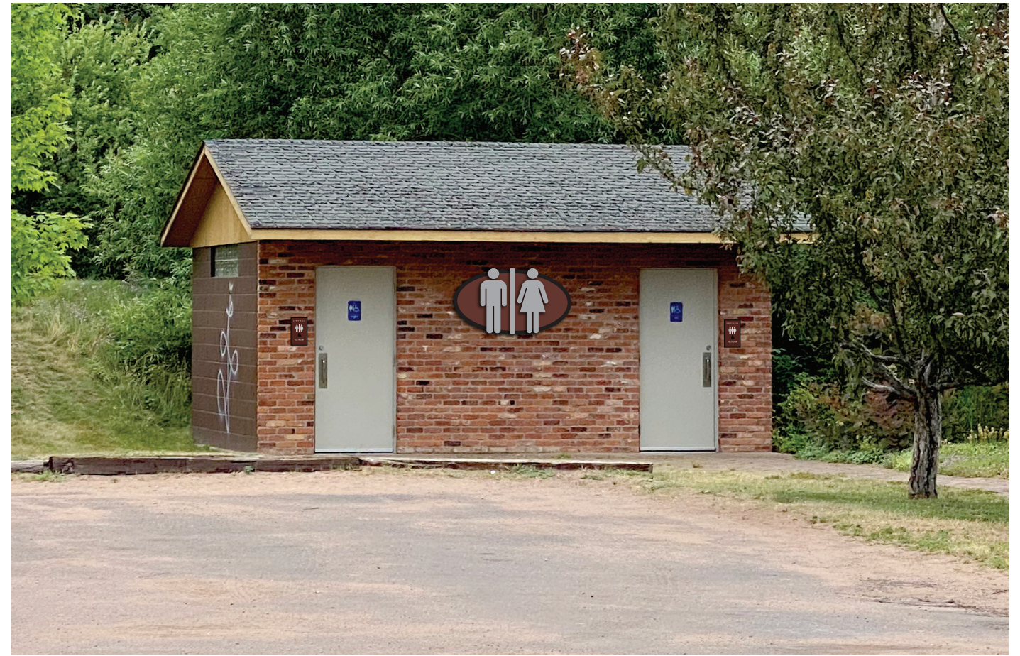
2 Photo Composite SCALE: NTS Front St Restrooms
